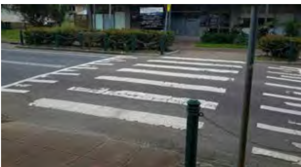
Non-compliant zebra crossing (no tactiles): ZC_00003
