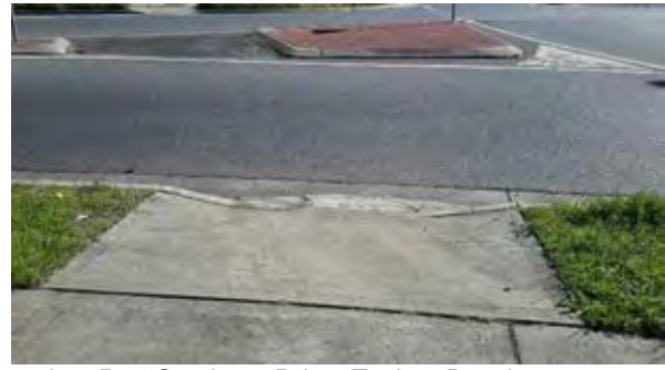
Visually DDA non-compliant kerb ramp: KR_00295
