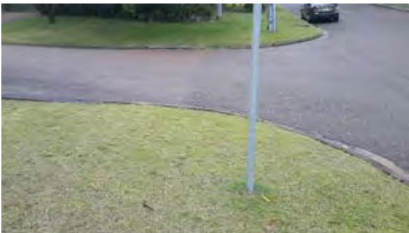
Missing kerb ramp: KR_00600
