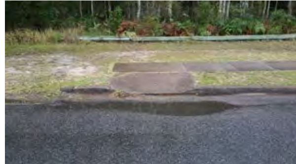
Visually DDA non-compliant kerb ramp: KR_00295
